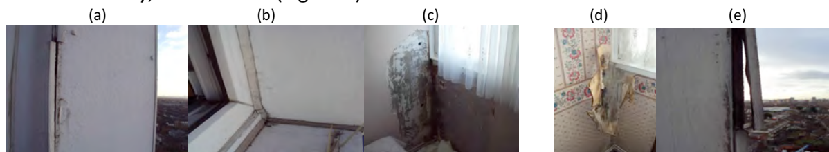
Figure 1. Damp and mould problems in Flat A (a, b, c) and Flat B (d, e) in the tower block in LBN
