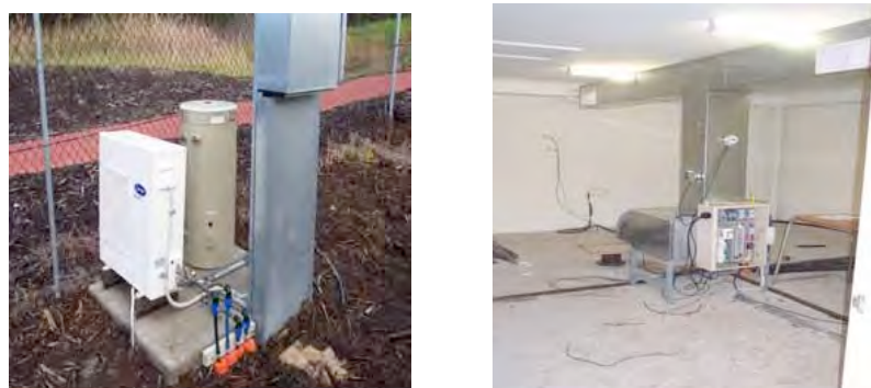
Figure 4. Water chiller (on left) and fan coil (on right) unit
