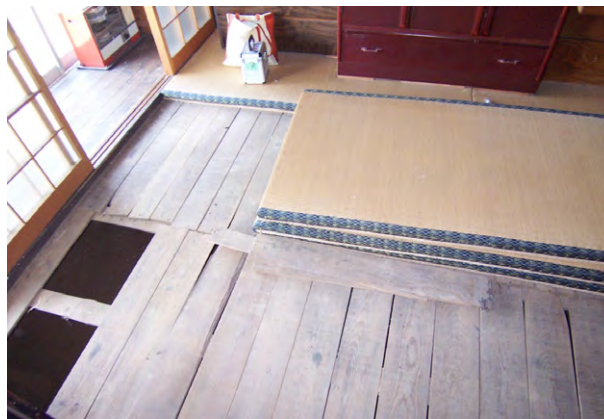
Figure 5. Damaged Tatami mats were reused for insulation. Less damaged floorboards were carefully removed and saved for exterior work.
