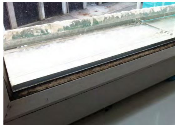
Figure 6 Occurrence of a severe mould growth problem on inside of windowsill
