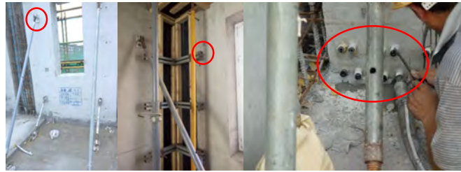
Figure 6. Bolt hole and grout hole.
