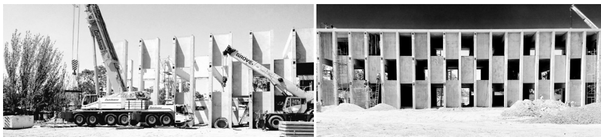
Picture 6. Construction and assembly of the structure and panels
