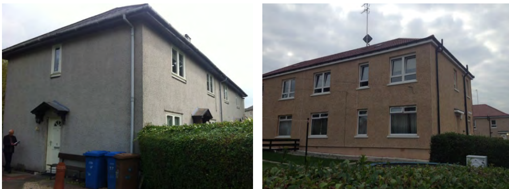
Figure 1 Typical uninsulated property (left) and externally insulated property (right)
