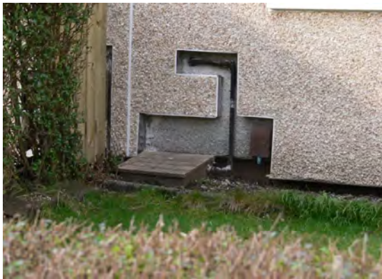
Figure 5 Thermal bridge due to non-insulated section around a gas pipe and meter box and meter box
