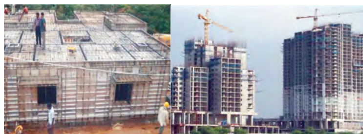
Figure 3: Monolithic concrete construction (Source: http://www.mhupa.com )
