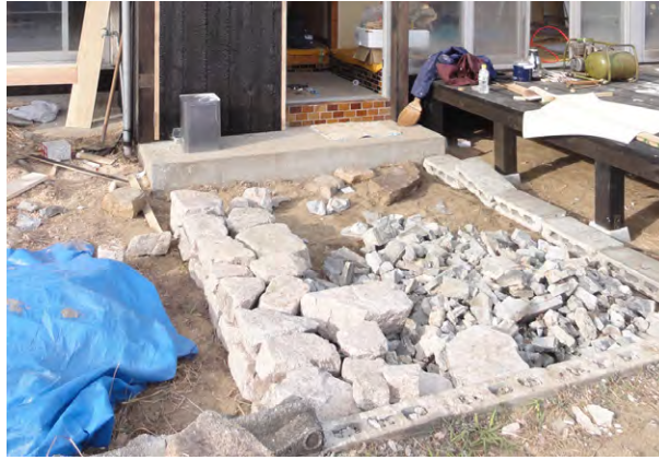
Figure 6. Concrete blocks were crushed and reused for the entrance approach.
