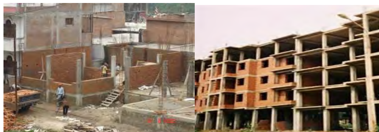
Figure 2: RC frame with brick as filler block (Source: http://www.world-housing.net )
